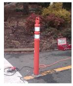
bollards will block the path of a vehicle and send a clear visual signal that vehicles are not permitted on the trail.
