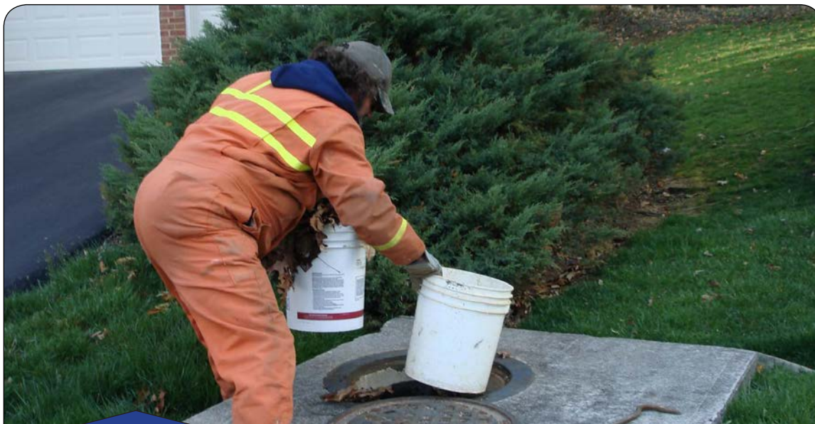
The Department of Public Works staff cleans out catch basins to help prevent nonpoint pollution.
