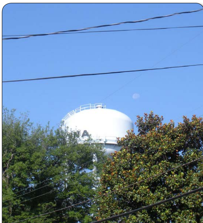
Several telecommunications facilities are located at a Vienna water tank on Tapawingo Road SW
