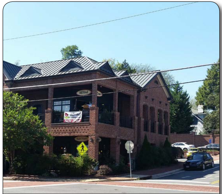
Street parking located on Church Street NW and Center Street N
