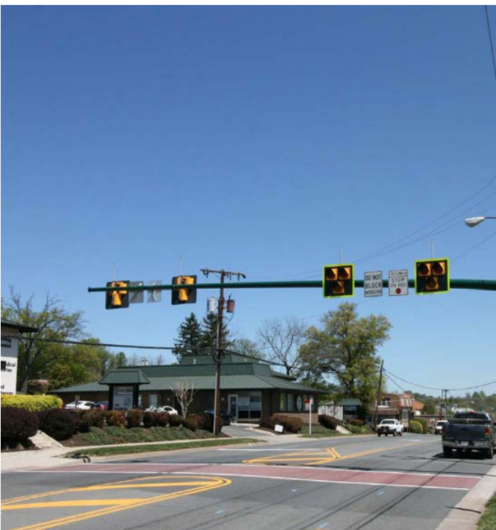
Pedestrian Signals: HAWK signal at the mid-block of the 300 block of Maple Avenue West
