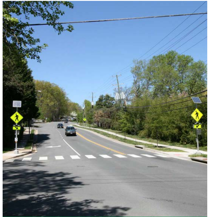
Hybrid Signals: Rapid flashing beacon at Lawyers Road and Blair Road NW
