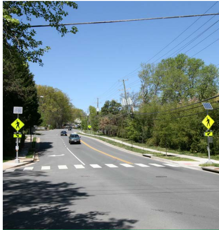
Hybrid Signals: Rapid flashing beacon at Lawyers Road and Blair Road NW
