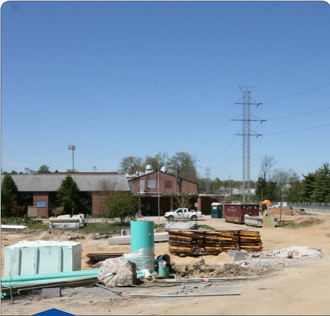
The Community Center is currently undergoing a complete renovation, along with the addition of a new gymnasium towards the rear of the building.
