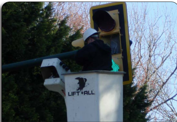
Vienna Public Works staff working on traffic signals
