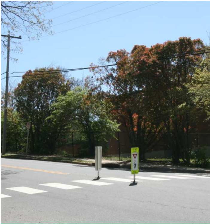
Signs: Pedestrian crossing signs at Marshall Road SW
