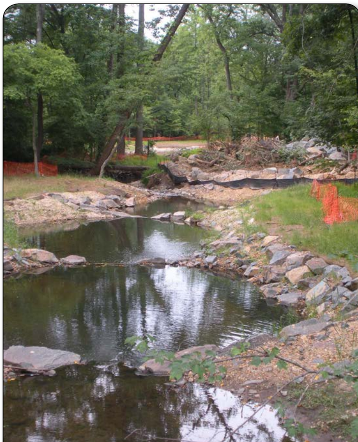
Wolftrap Creek restoration project near Follin Lane NE
