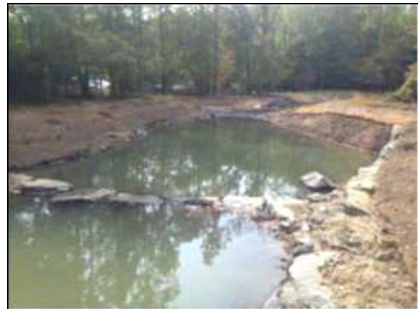
Wolftrap stream restoration during construction.
