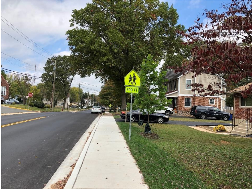
PHOTO 2A- NUTLEY ST NW- AFTER
