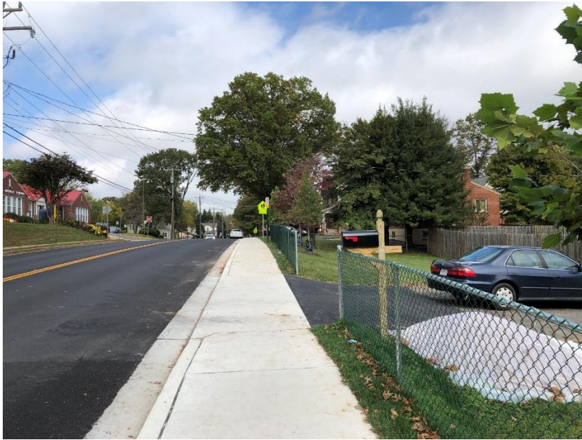
PHOTO 1A- NUTLEY ST NW- AFTER
