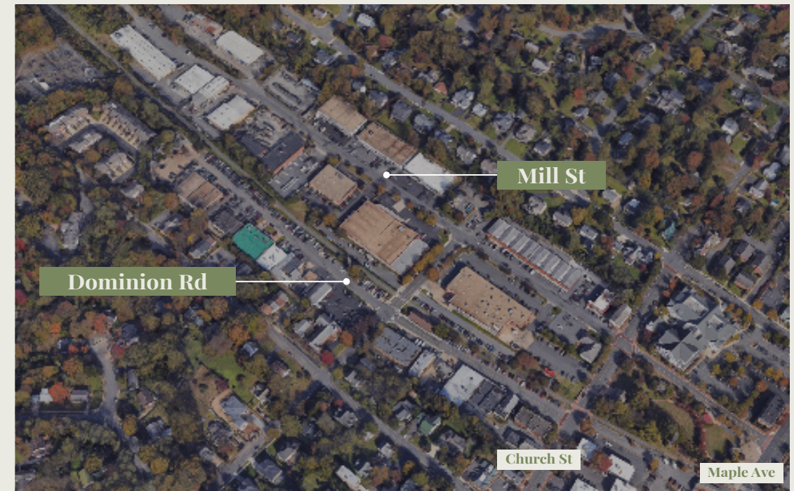
Aerial view of Mill and Dominion - limited sidewalk infrastructure in the commercial node owing to its history as an industrial-only zone.
