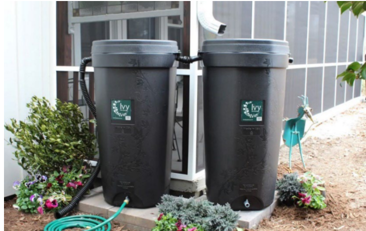
Rain Barrel System Collecting Runoff from Downspout (©Rain Water Solutions photo courtesy of the Metropolitan Water Reclamation District of Greater Chicago)
