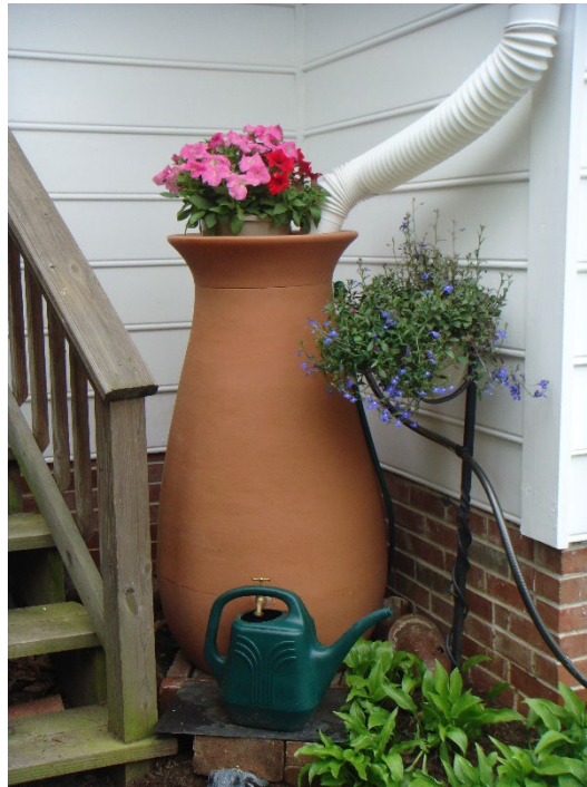
Rain Barrel Collecting Runoff from Downspout (Photo courtesy of the City of Rockville)
