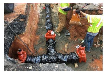
and property owners and residents are notified. For out-of-town work, special permits are required from VDOT. Work begins when existing utilities are marked, and pipe locations are verified. Water services, gas services, buried electric lines, and fiber optic cables all must be carefully protected from damage via a hand digging process. Construction crews then replace existing 4" thru 8" cast iron water mains with new concrete lined ductile iron water pipes.
