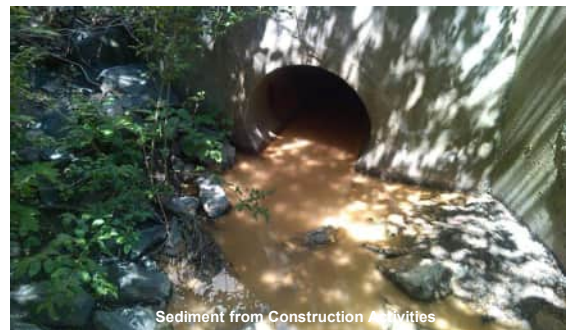
Sediment from Construction Activities
