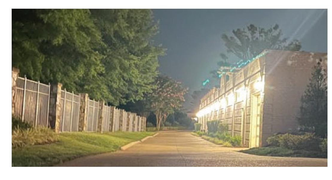
The photo above shows high-glare wallpacks being used for security lighting. While it is important for public safety to have enough light near exits and on the driveway surface, there is a lot of light in the trees, passing the fence, and in our eyes.
